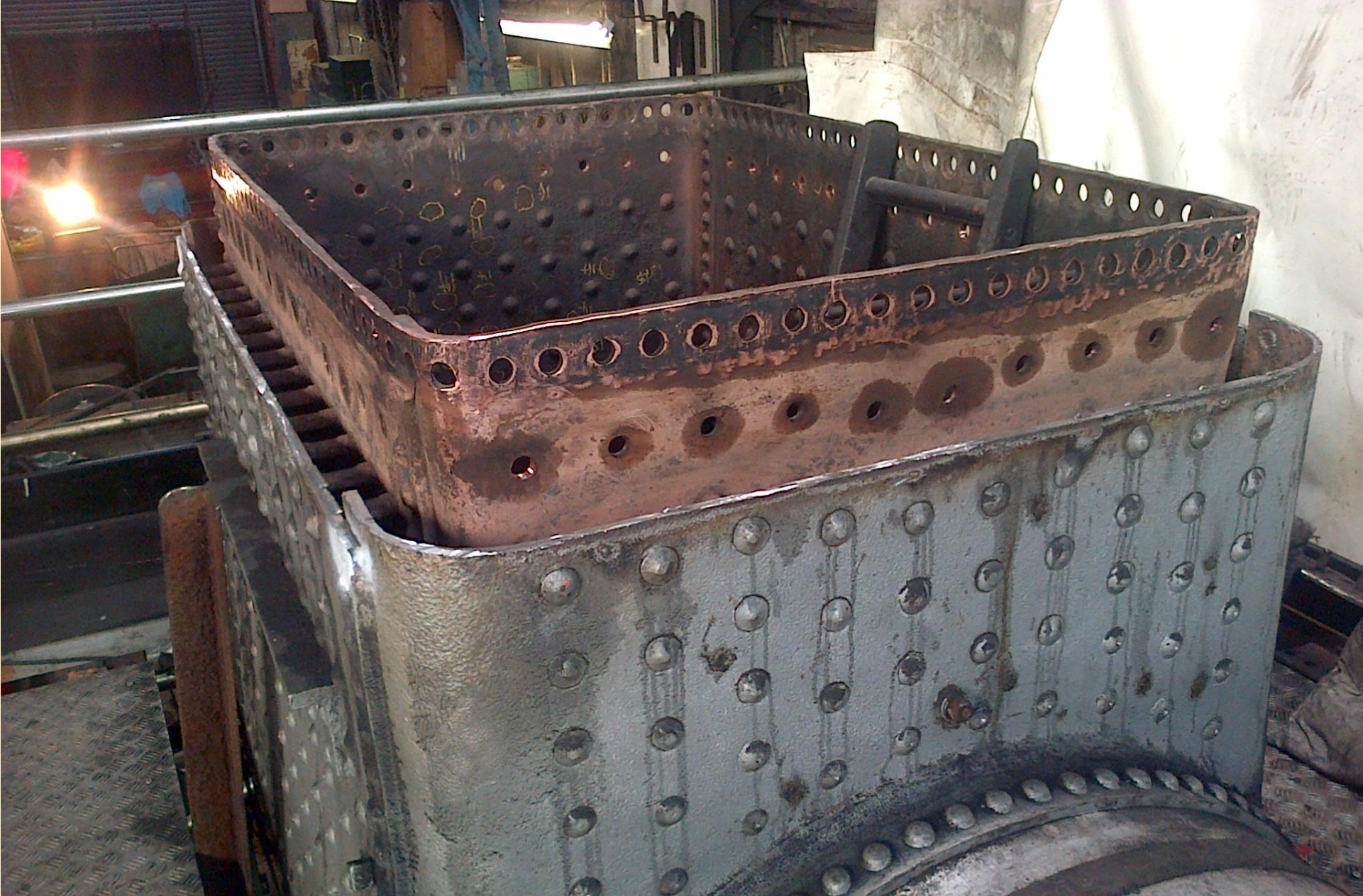
Defective Plate removed. Loco 25
